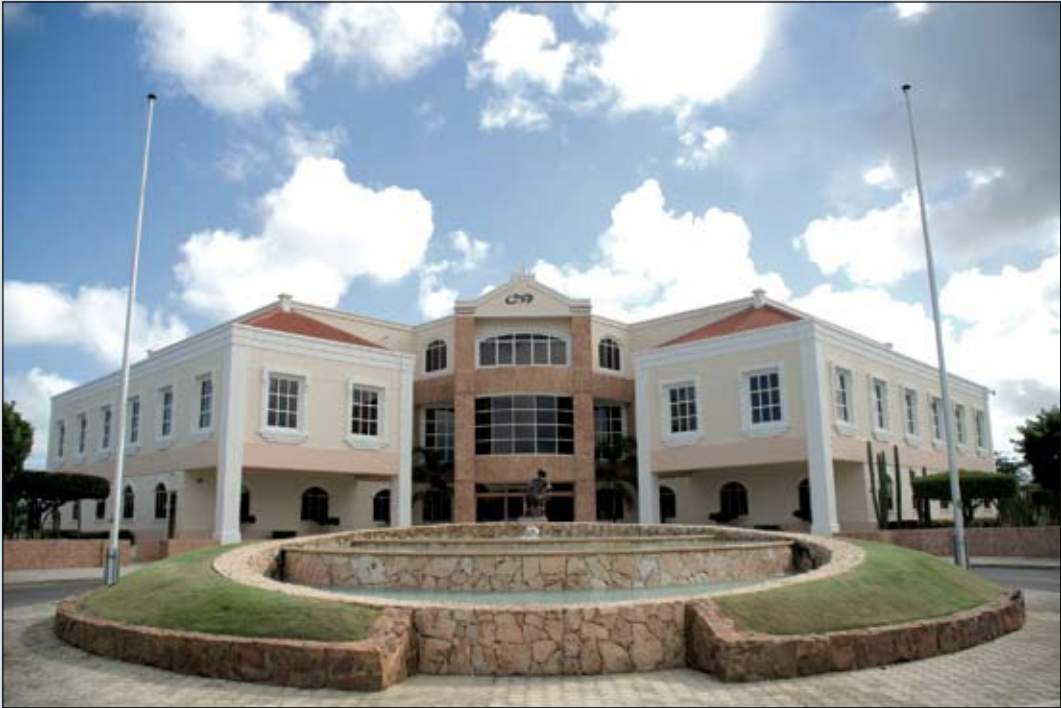
The office building of the CBA at J.E. Irausquin Boulevard 8
